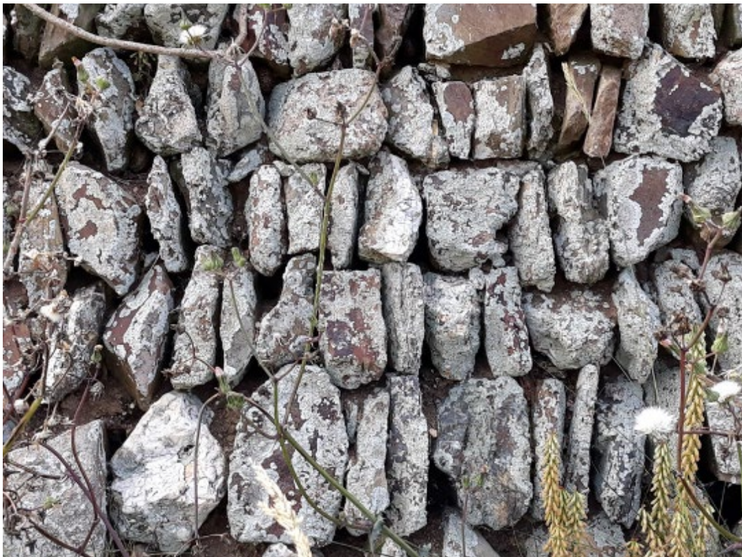
Figure 13: typical stone facing to Cornish hedges in the Undulating Land Type (credit LLCA Team)
