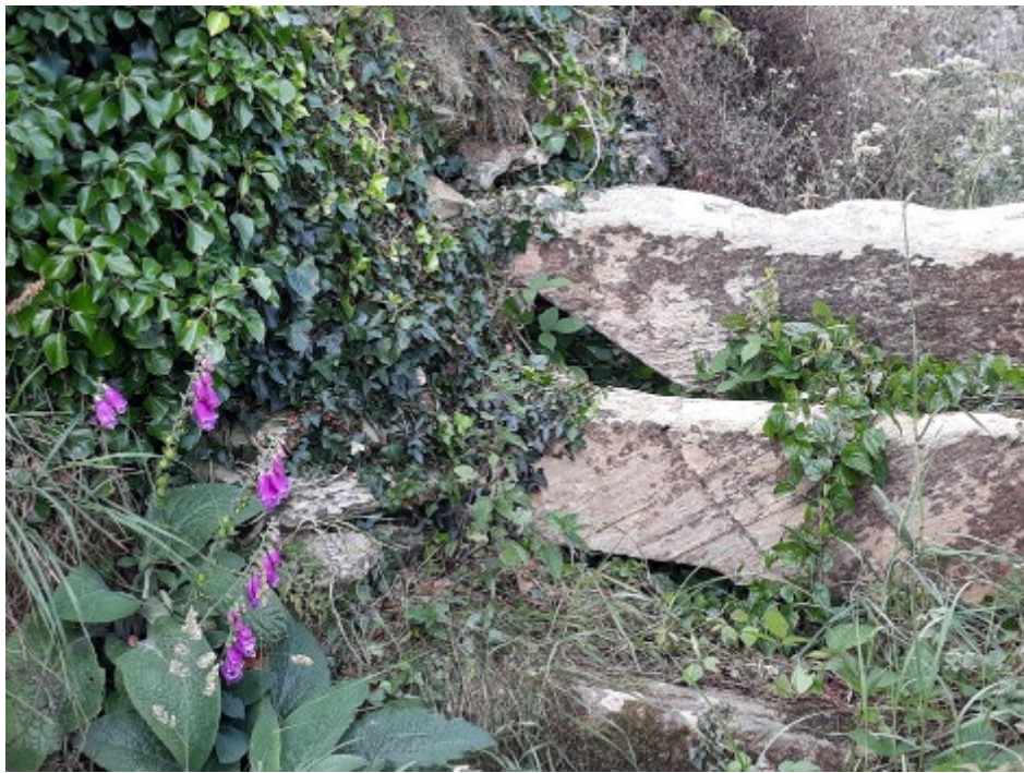
Figure 17: Example of historic step made of locally-sourced stone over stile on footpath near Lambourne Farm, Penhallow (credit LLCA Team)
