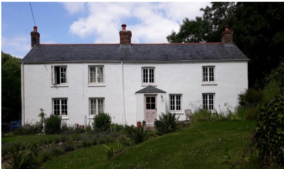
Figure 31: Swallowfields, Penwartha, a typical cottage dating from the 1770s built of local quarry stone and cob with slate roof and a later (early C20 addition) in a style sympathetic to the original (credit LLCA Team)
