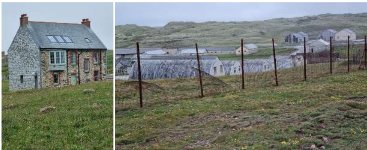
Figure 45: Renovated former Mine House at Penhale and huts of Penhale Camp (credit Philip Henwood)
