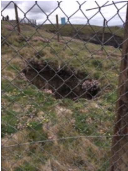
Figure 41: Fenced open mine shaft at Cligga (credit LLCA Team)
